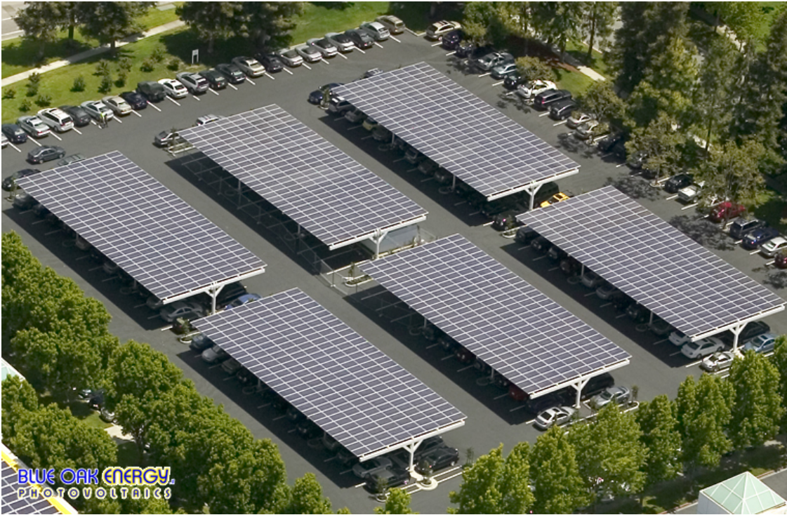
Photo credit by Blue Oak Energy Photovoltaics
